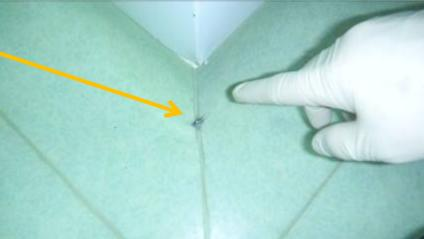
Difficult to clean, corrosion leads to particle release
